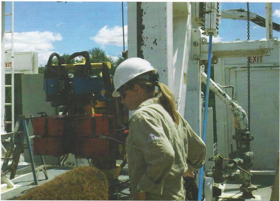
DEQ-OOGM Geologist inspecting floor of rig during drilling operation.
